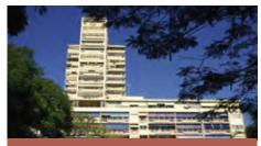
Torbreck Home Units in Highgate Hill, Brisbane, was erected in 1958-1960 in two sections: an eight-storey garden block to Chermside Street and a fourteen-storey tower fronting Dornoch Terrace. The eight-storeyed garden block was constructed using the lift-slab technique: the roof and floors were prefabricated in concrete on the ground, then hoisted into position by jacks mounted on the vertical wall supports. This was the first use of this construction technique in Queensland.
