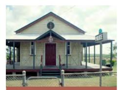
The **Police Station and Courthouse** (former) at St Lawrence was constructed in 1878. As a single-storey, single-skin timber, government-designed building, it is significant as a rare surviving and highly intact example of a type of courthouse/police station design and construction once common in Queensland. Few early timber police station and courthouse buildings survive and the St Lawrence building has rarity value as one of the earliest, intact, extant examples of its type.
