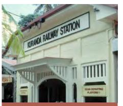
The **Kuranda Railway Station** in far North Queensland, erected 1913-1914, is an early example in Queensland of pre-cast concrete construction utilising a system of reinforced concrete planks slotted horizontally into a concrete frame supported on in-situ concrete dwarf walls. It is one of the earliest railway stations to be built in Australia using standard pre-cast concrete units and the oldest remaining example of its type in Queensland.
