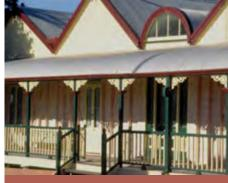
The **Pfeiffer House**, Charters Towers, was built c1881 for local mining magnate Frederick Pfeiffer. The place has rarity value as an early example of exposed timber stud construction in North Queensland and has an unusual form. It also demonstrates a way of life no longer common, being built near the entrance to Pfeiffer's former mine. The practice of positioning a manager's or owner's house in close proximity to a factory, mine or mill is no longer common.
