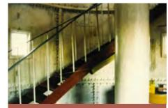
Bustard Head Lighthouse (1868) was the first lighthouse built by the Queensland colonial government. It remains highly intact and is important in illustrating a construction technique using bolted prefabricated segments of cast iron imported from England. It is one of only two prefabricated cast iron lighthouses erected in Queensland, the other being the Sandy Cape Lighthouse, constructed in 1870.
